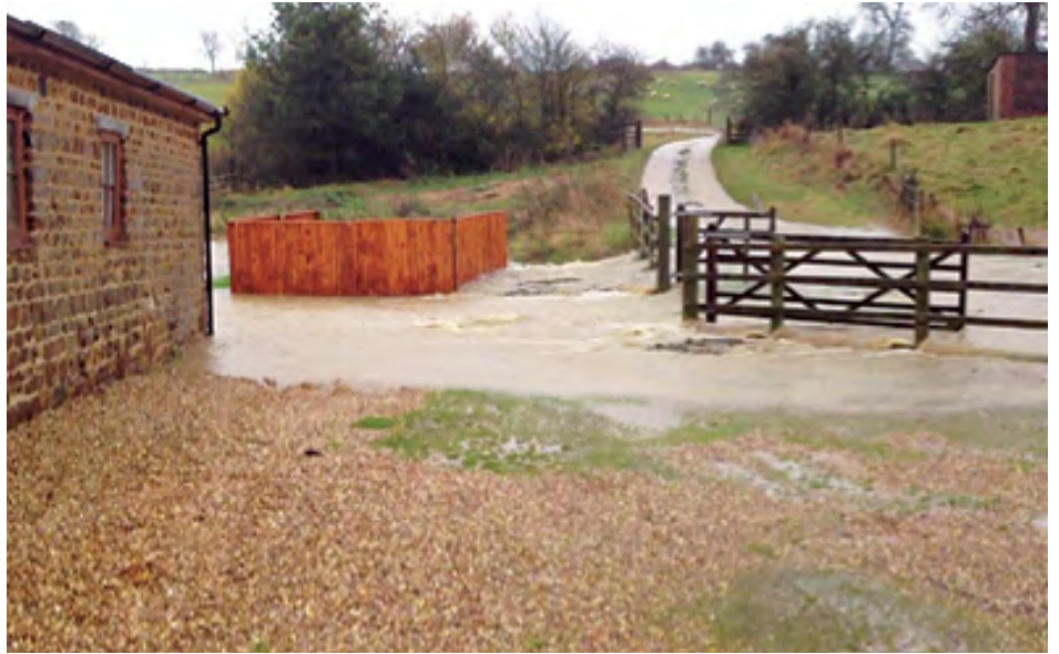
Flooding at The Granary Hotel.
