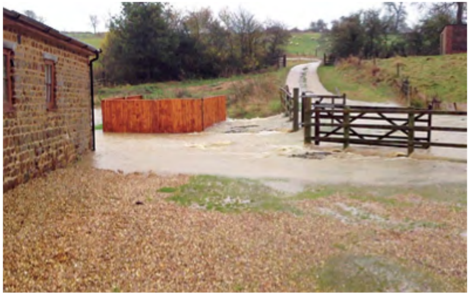
Flooding at The Granary Hotel.
